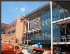
West Elevation Glass Curtain Wall.
