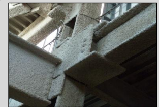
Column-to-beam moment connection.
